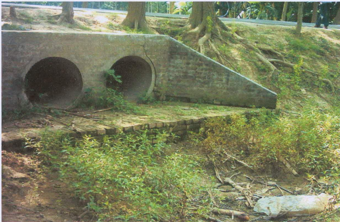
Plate 10: A tunnel for drain off water
