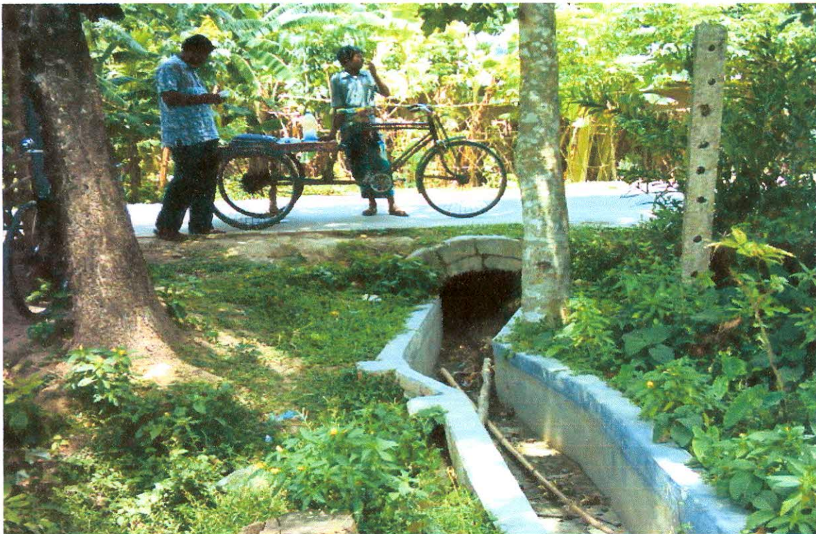
Plate 21: Under-pass irrigation channel that can be adopted; not cutting road and embankment
