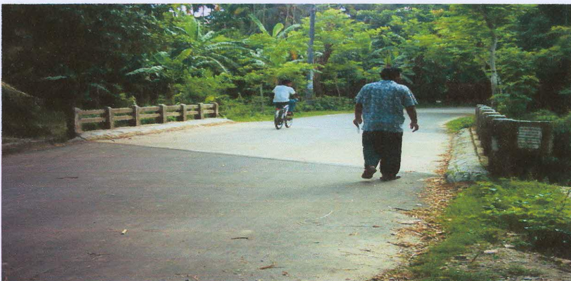
Plate 14: Culvert constructed by LGED and CARE in 1995
