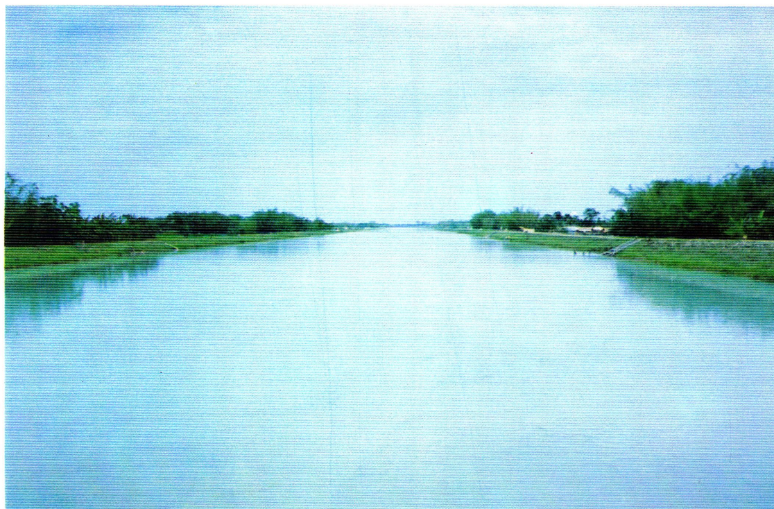
Figure 1.5 Teesta Main Canal
