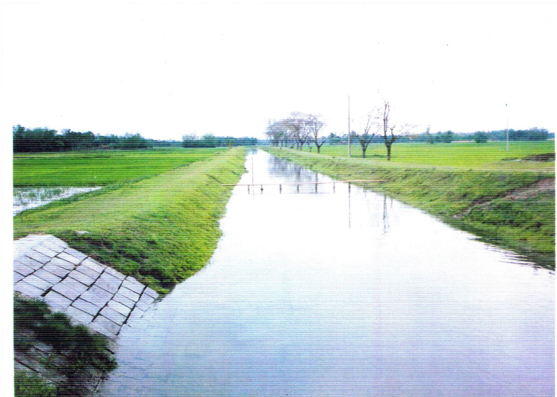
Figure 1.6 Tessta Project Secondary Canal
