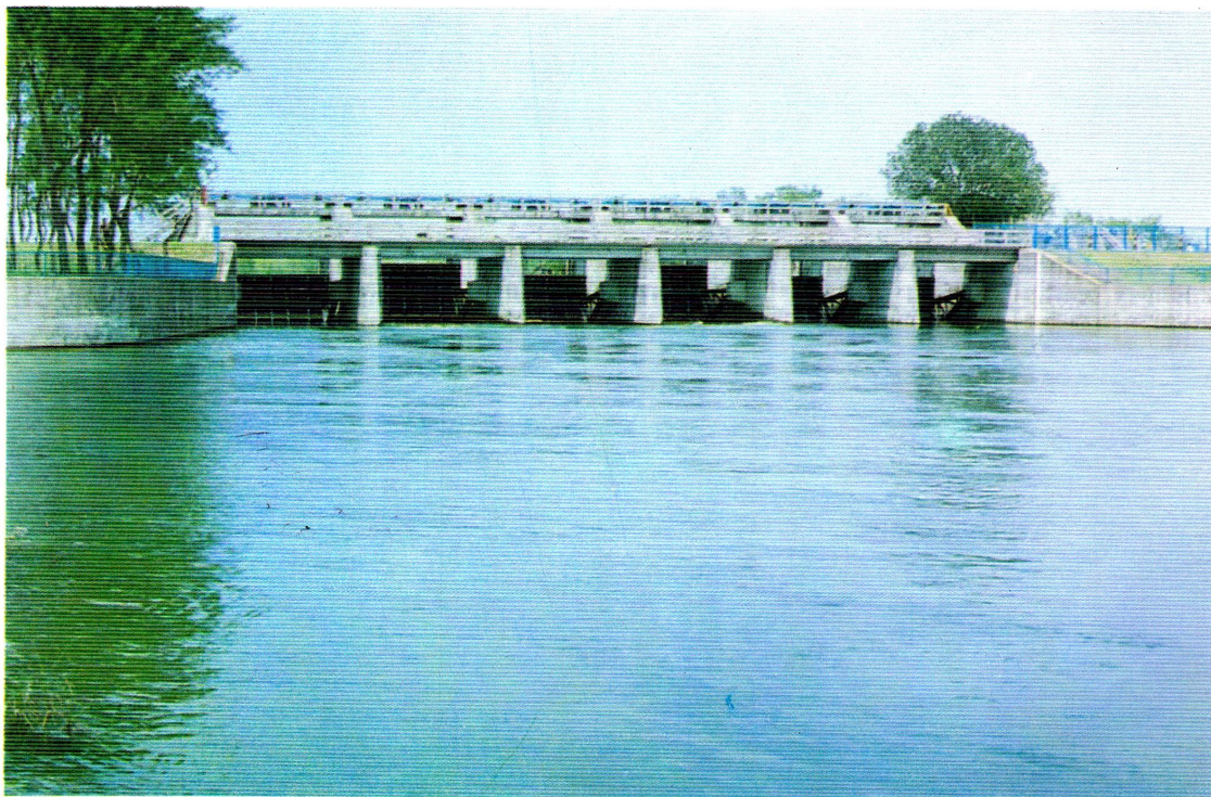
Figure 1.4 Teesta Project Main Regulator
