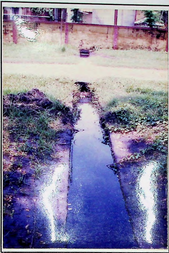
Photograph 5- Effluent Discharge Drain of the Sugar Mill.
