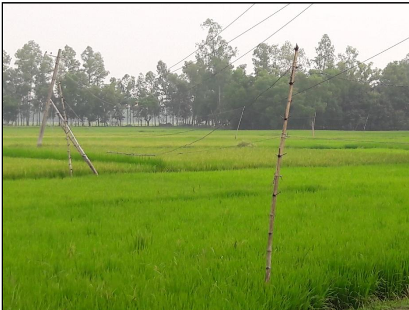
Figure: 6.4: A view of electric wire was pulled by bamboo in the study area.
