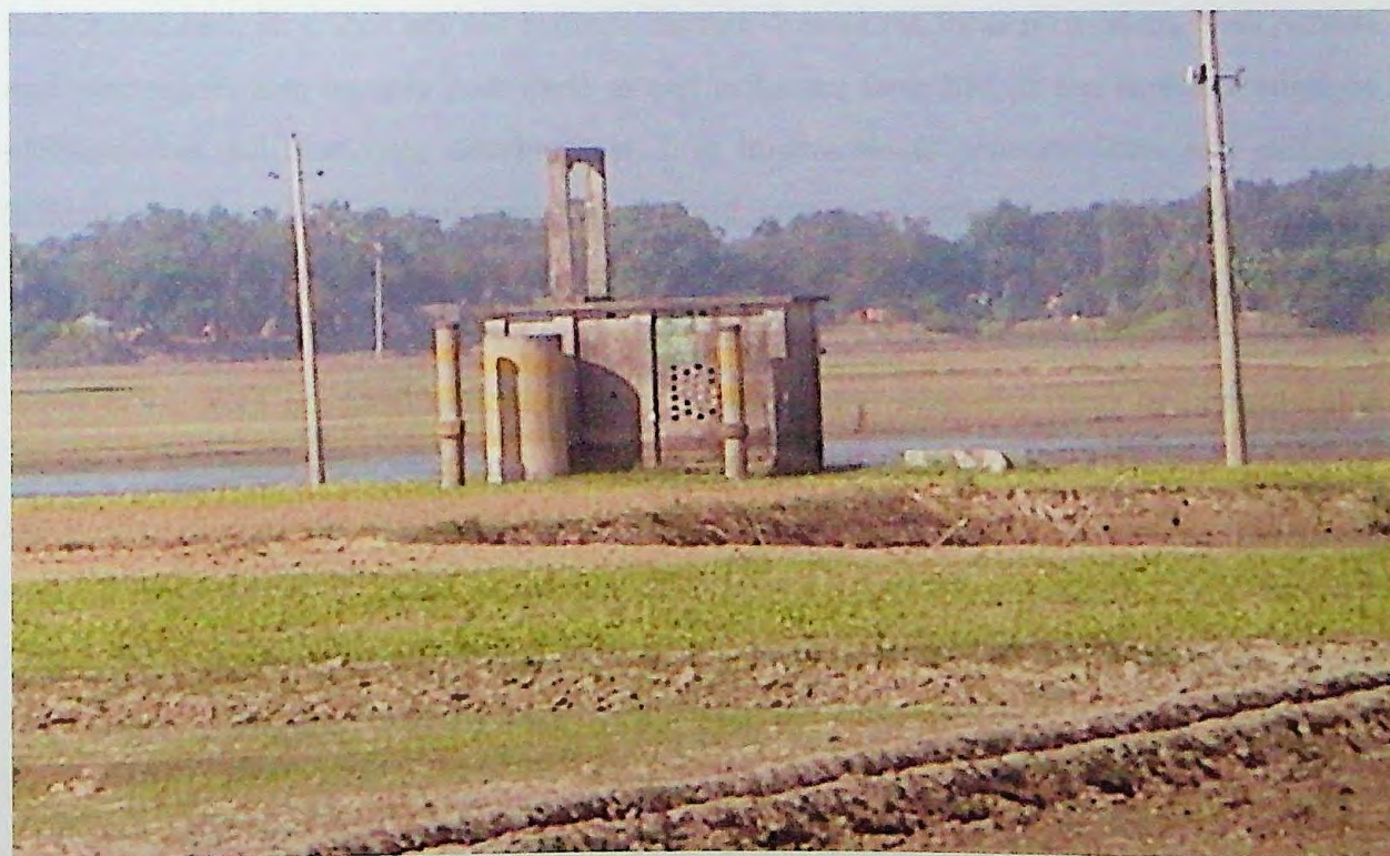
Fig. 4.21 Irrigation controlled by Deep tube well (Ground water) in the study area in recent years
