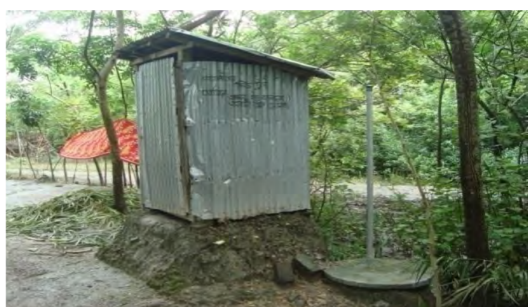
Raised Platform of Sanitary Latrine and Community Tube well in Khurushkul Union (Source: Field survey, 2016)
