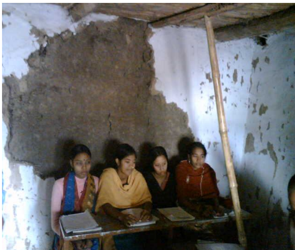
Picture 4.3 Infrastructure of Kamargaon High School (Class room)
