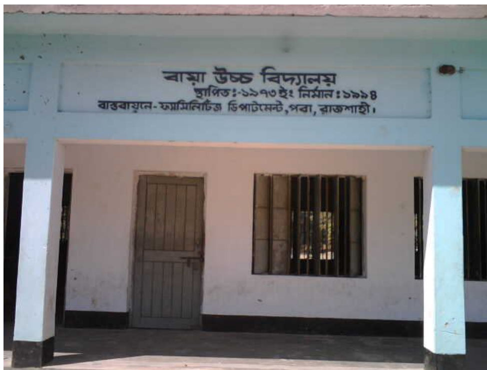
Picture 4.6 School Building of Baya High School, Rajshahi
