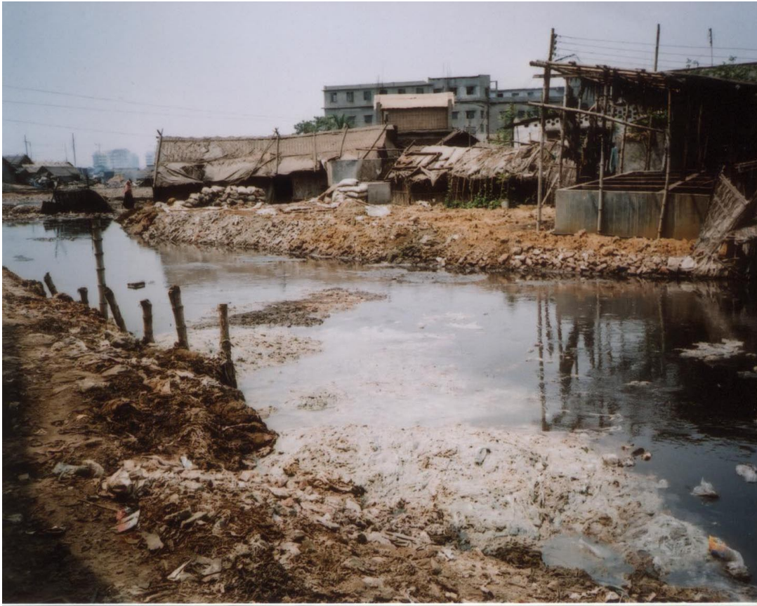
Photograph -12: Fleshings & other Solid Wastes reducing the carrying capacity of Hazaribagh_Canal near Kalunagar at Hazaribagh
