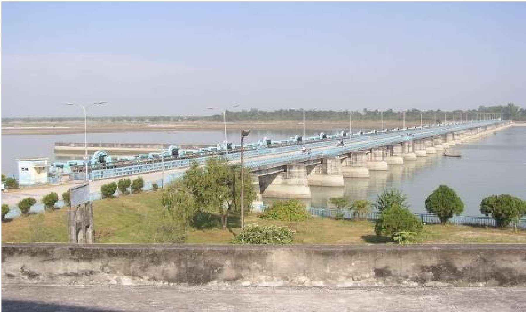
Figure 1.2 Photograph of Teesta Barrage
