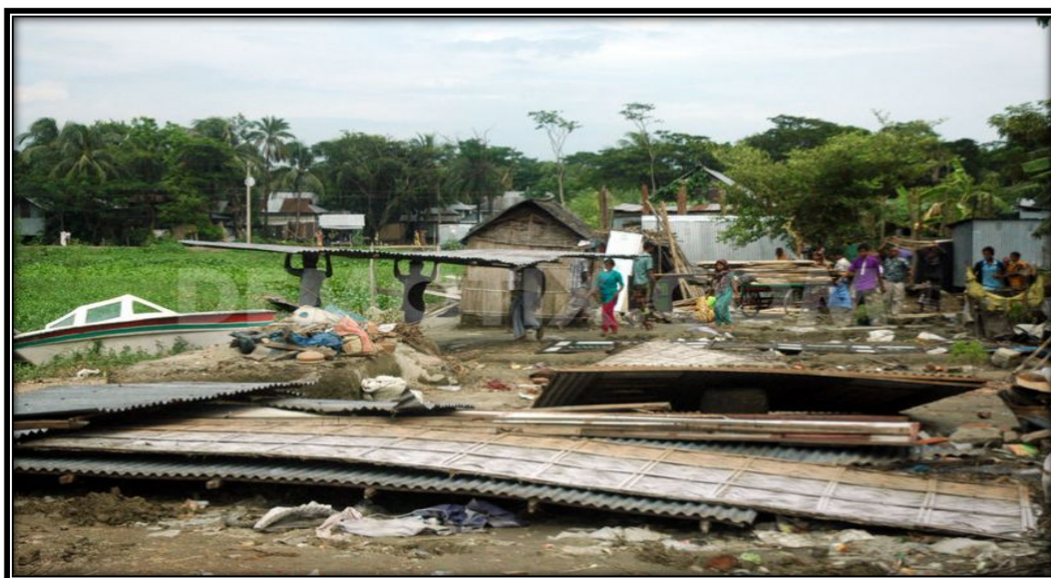
Photo 6.2: Shifting of Housing structure
