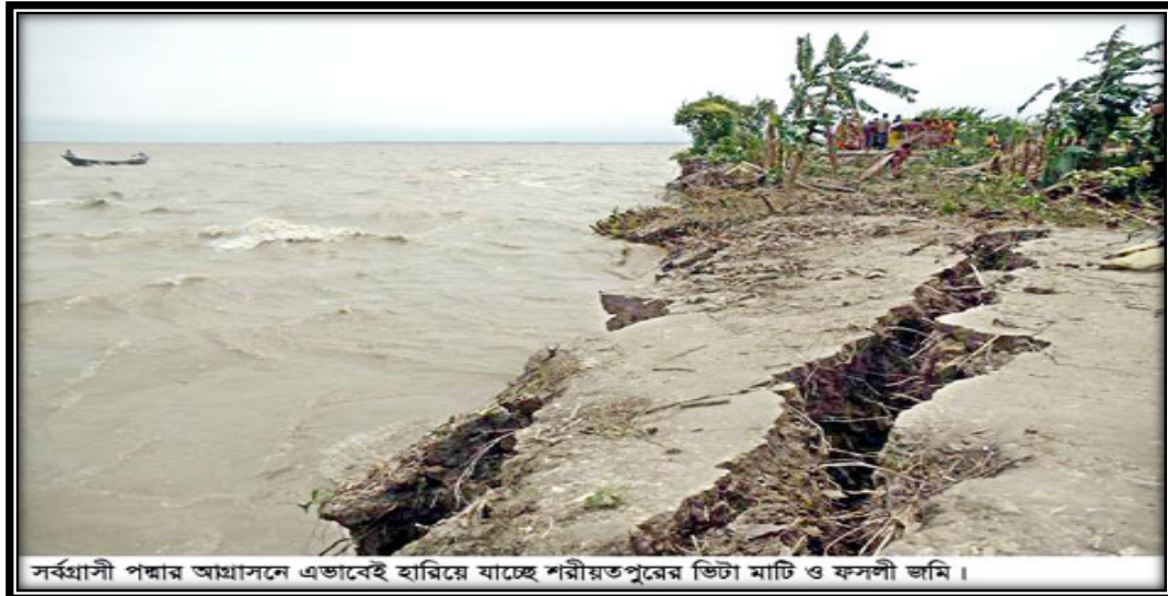
Photo 3.2. Erosion at Shariatpur
