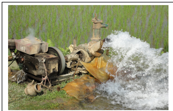
Photo-1: Shallow Pumps in Sirajganj
