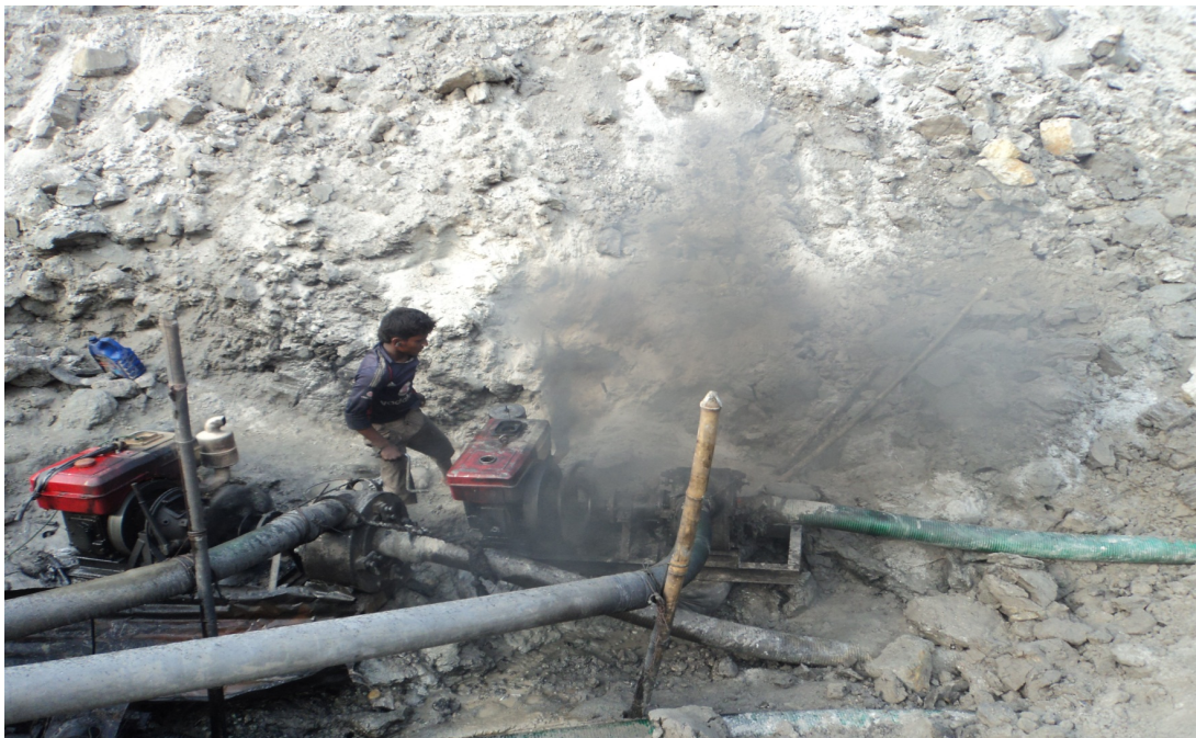
Picture 5: Use of Machines for Removing Water from the Stone Quarry
