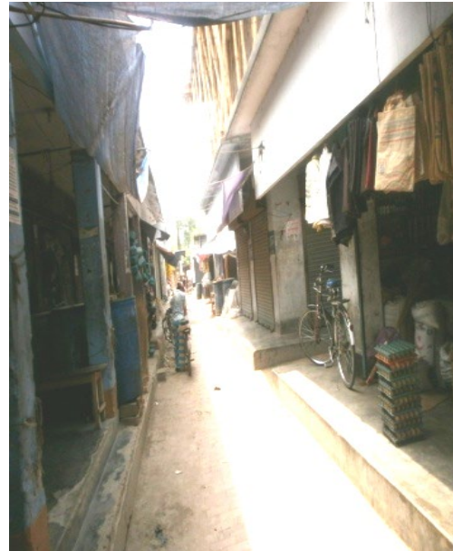
A One Story Building at the Market
