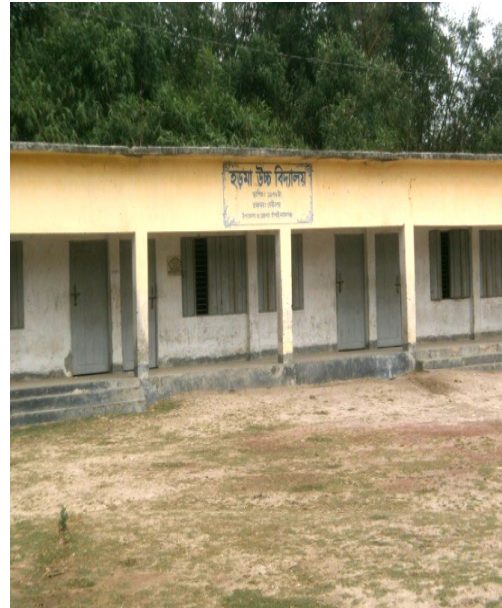
A primary School at the Premises of the Haat
